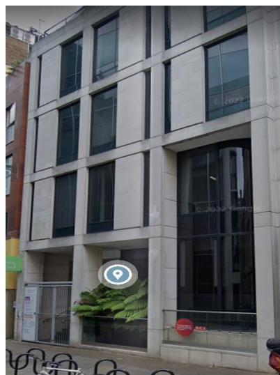
View of entrance looking north (from Whetstone Park corner)
