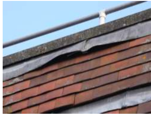
Figs. 21 & 22 Gaps behind lead flashing
