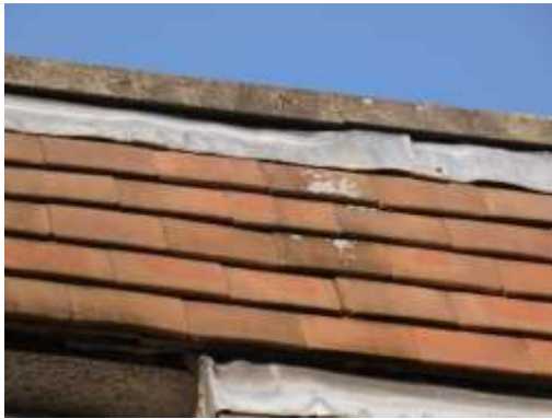
Figs. 21 & 22 Gaps behind lead flashing
