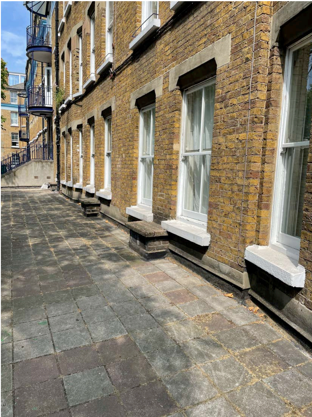
Fig. 02 Existing basement vents to be demolished and ground surface pressure washed & made good for re-use in other parts of site
