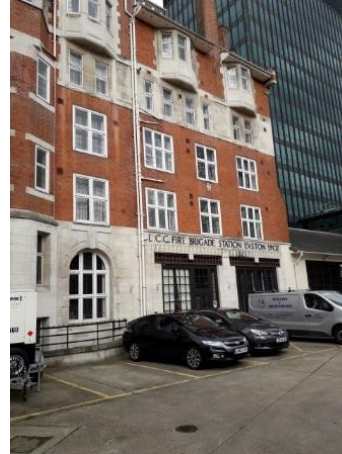
Photograph 02 – Euston Fire Station
