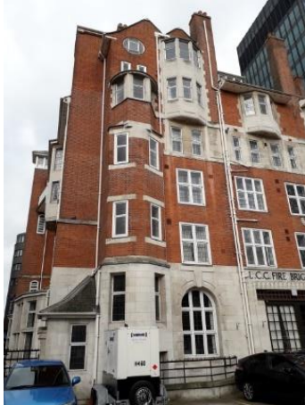
Photograph 01 – Euston Fire Station
