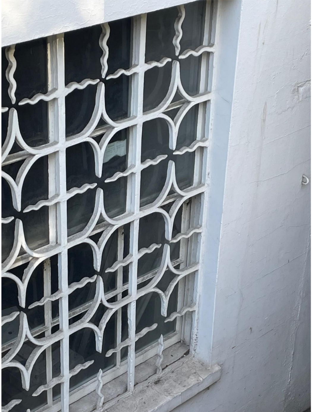
Type 3 surround square bar fixed by square bar spigot into reveal
