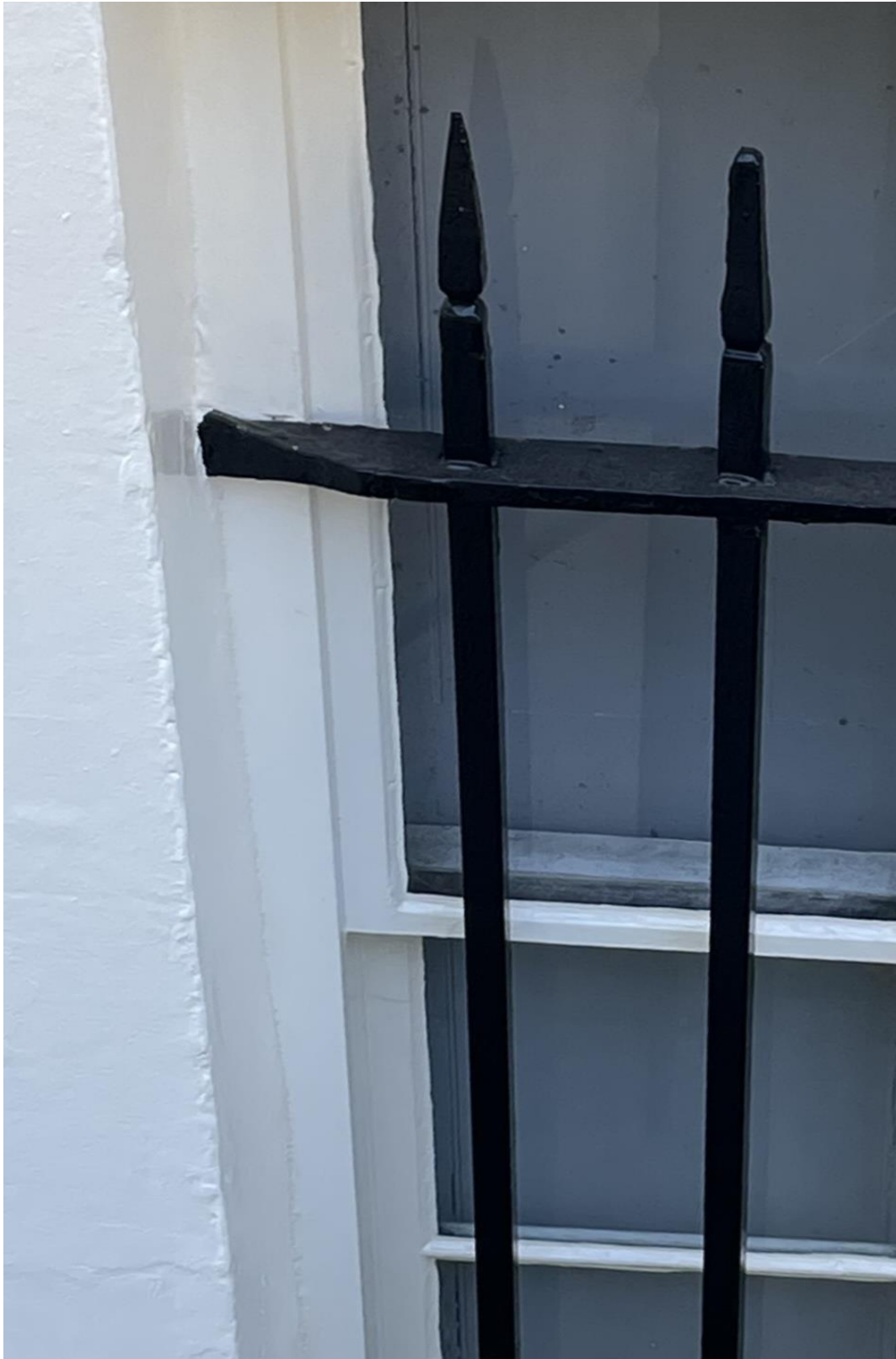
Type 4 horizontal bar forged to vertical lozenge into reveal.
