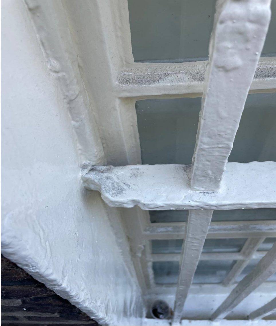
Type 1 diamond/square bar spigot into reveal
