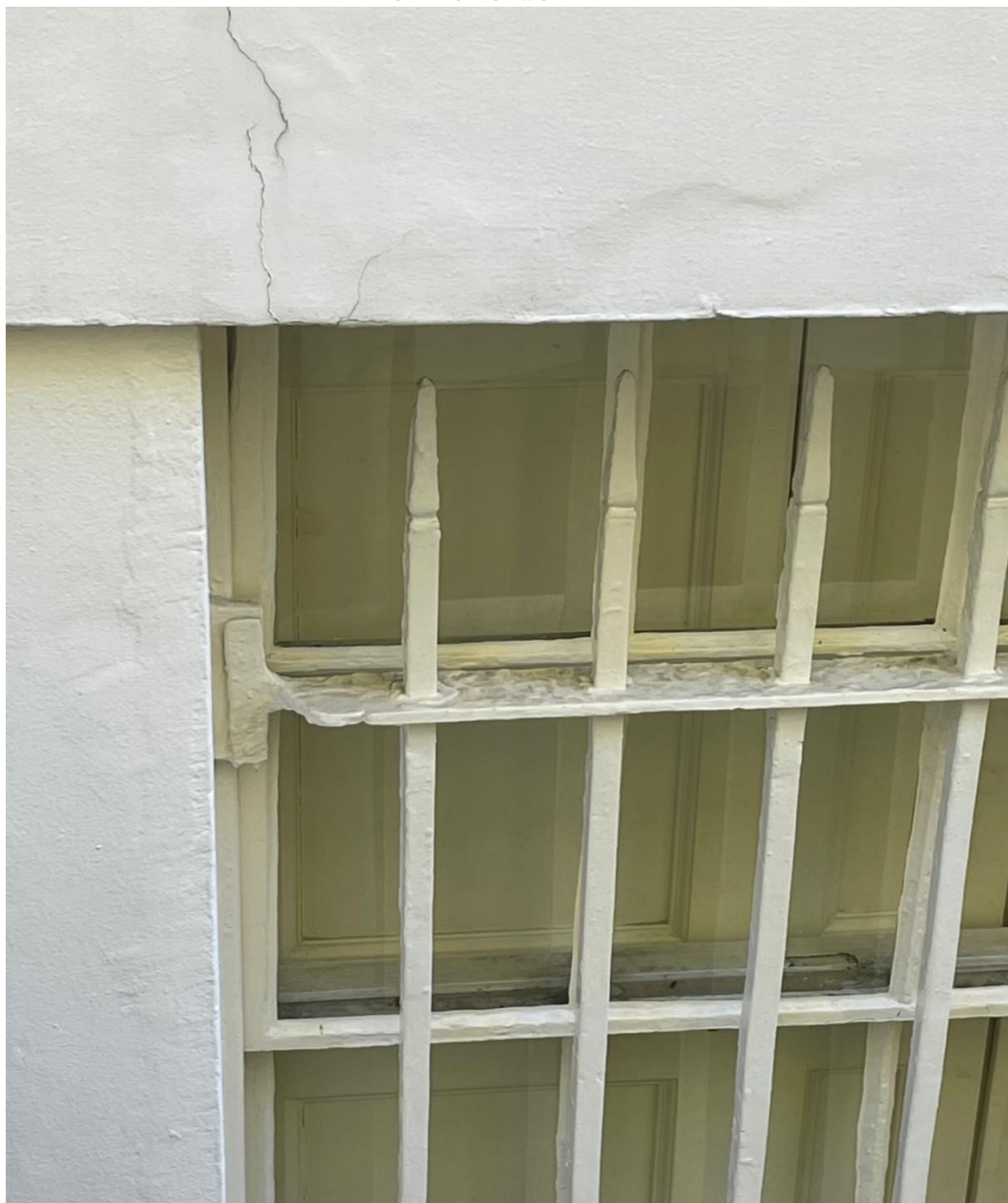
Type 2 bracket fixing to reveal
