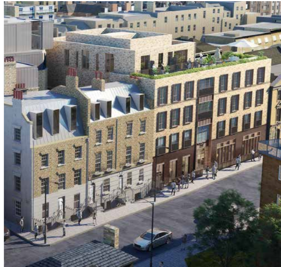
7abc Bayham Street (Hotel) Exterior
