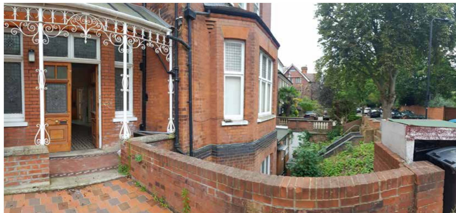
FIG. FRONT LIGHTWELL BOUNDARY WALL - IMAGE 03
