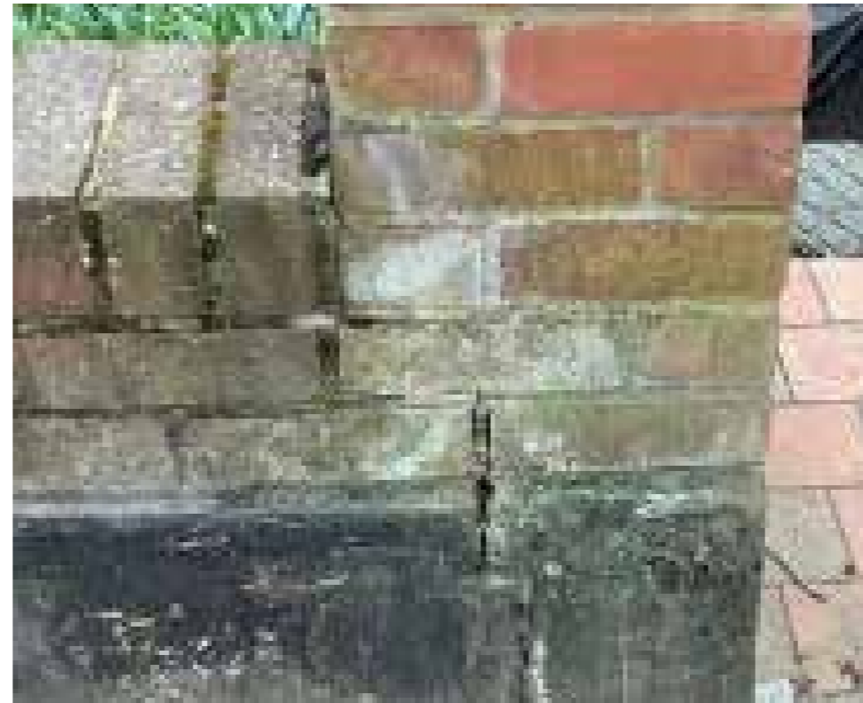
THE WALLS ARE CRACKING AND THIS IS LIKELY TO BE RELATED TO THIS GROWING TREE. CRACK REPAIRS TO THE WALL ARE NEEDED.
