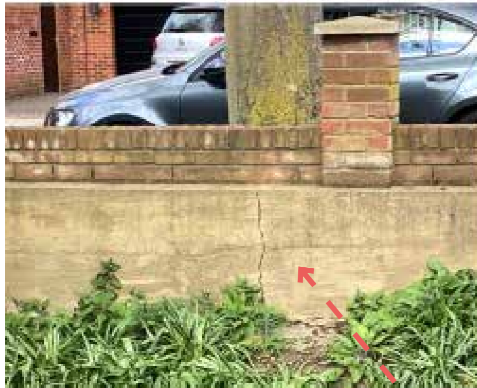
THE WALLS ARE CRACKING AND THIS IS LIKELY TO BE RELATED TO THIS GROWING TREE. CRACK REPAIRS TO THE WALL ARE NEEDED.
