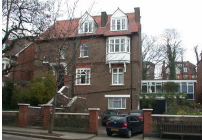
Image – photograph of the existing building as viewed from the street
