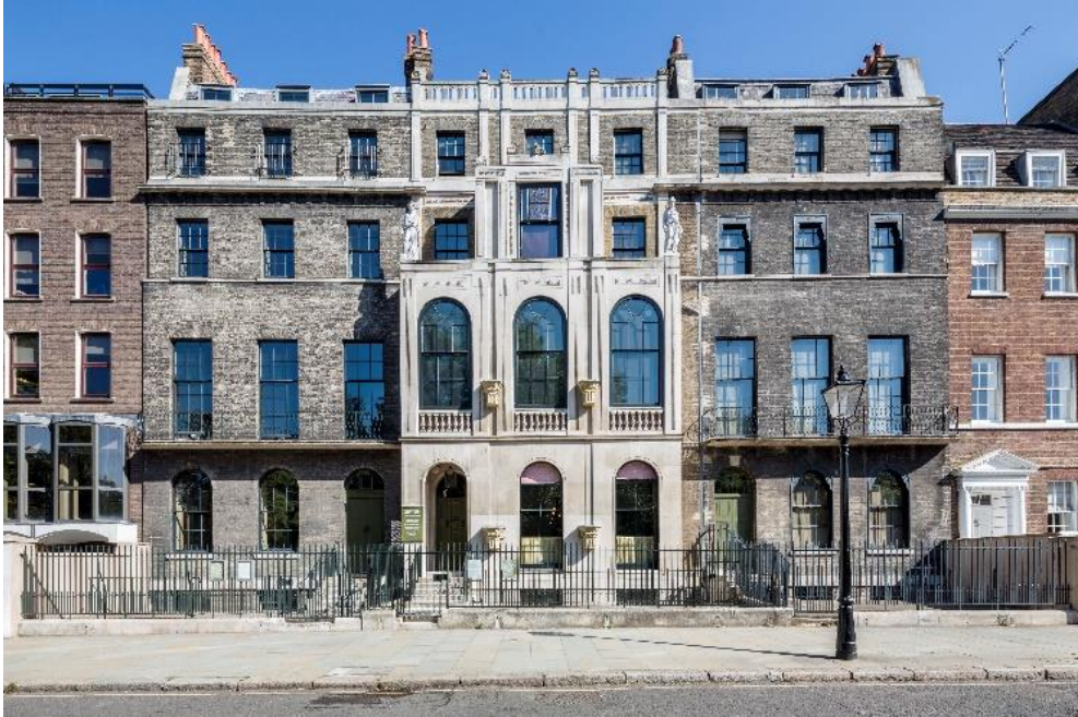
1. Front elevation view of site and neighbouring buildings
