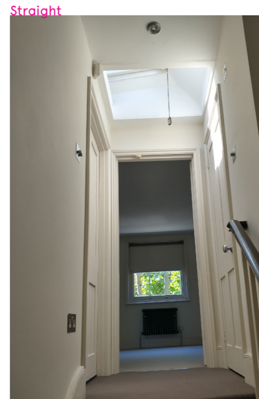
Third Floor Skylight
