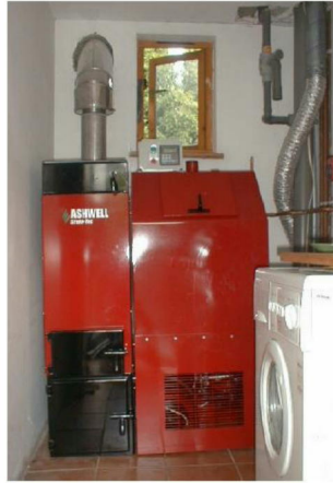
Figure 8 - Typical Biomass Boiler showing adjacent fuel hopper
