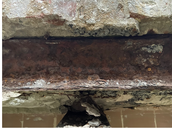
Existing overhead structure in the storage area: large parts of the steel sections have been lost, and delamination is occurred throughout. Additionally, the concrete has spalled due to the corrosion expansion.
