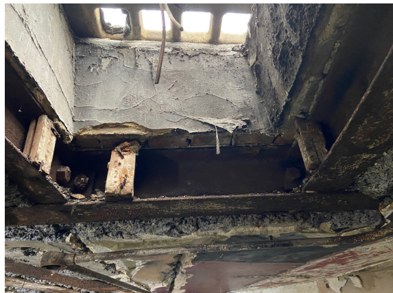
Existing overhead structure in the storage area: large parts of the steel sections have been lost, and delamination is occurred throughout. Additionally, the concrete has spalled due to the corrosion expansion.
