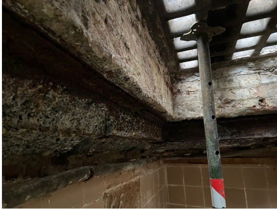
Existing overhead structure in the storage area: large parts of the steel sections have been lost, and delamination is occurred throughout. Additionally, the concrete has spalled due to the corrosion expansion.
