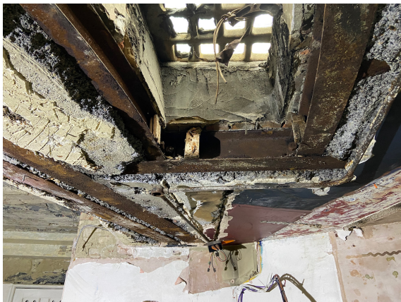
Existing overhead structure in the storage area: large parts of the steel sections have been lost, and delamination is occurred throughout. Additionally, the concrete has spalled due to the corrosion expansion.
