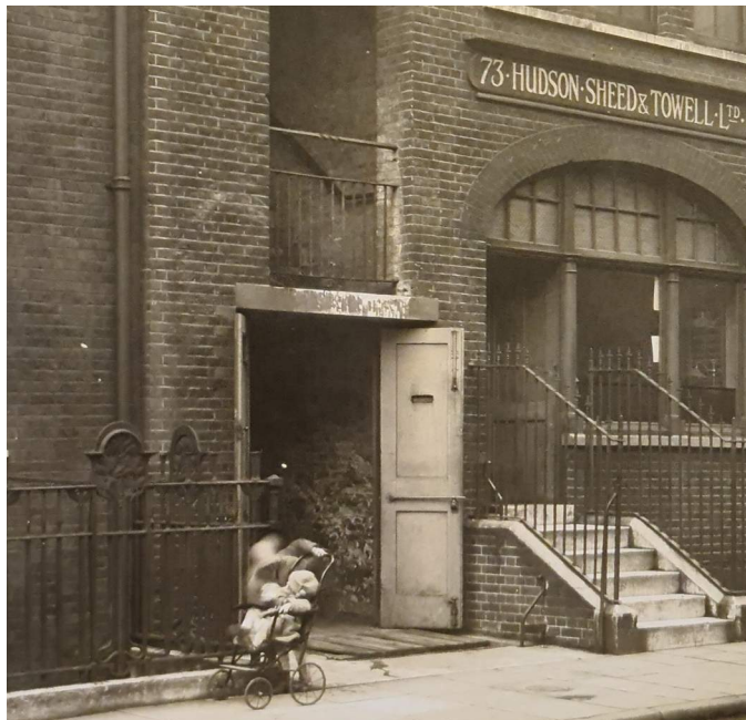
Fig. 8. Original Door at 73-75 Kenton Street
