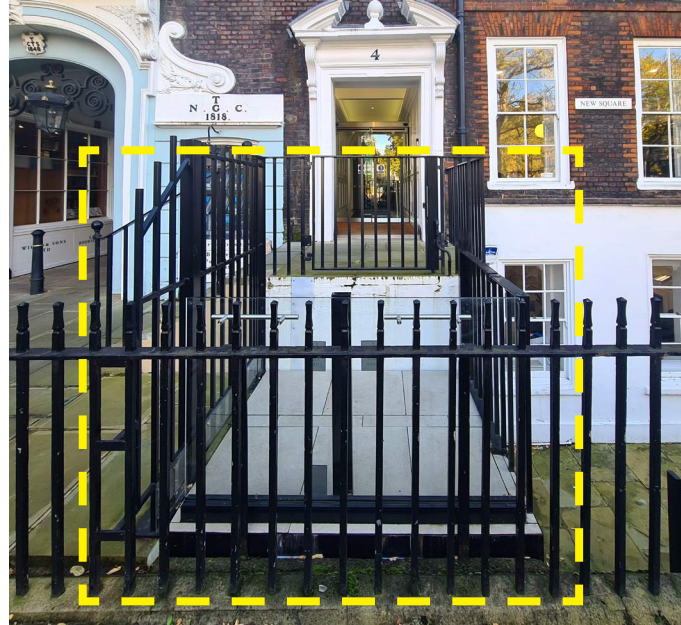
Fig. 15. 1 New Square with external platform lift
