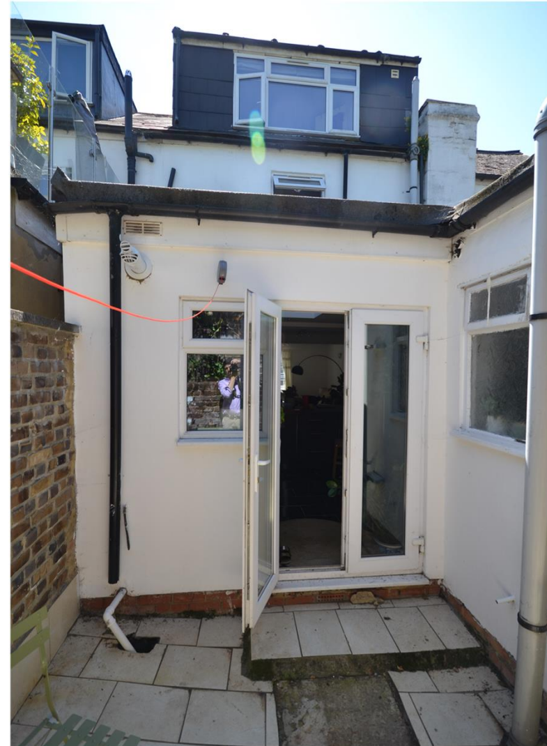
3. View of the rear elevation / location of new extension
