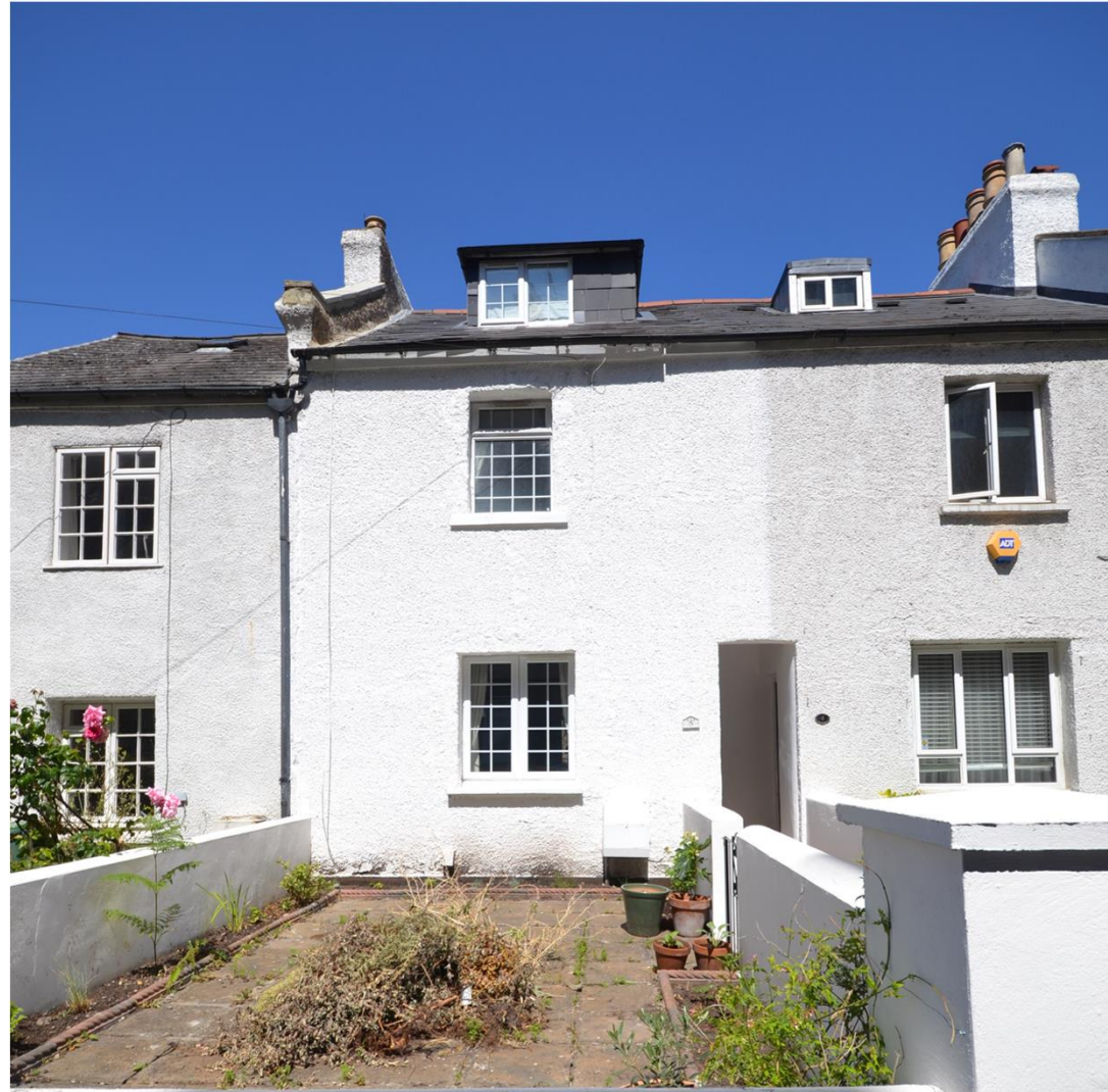
2. View of the front elevation
