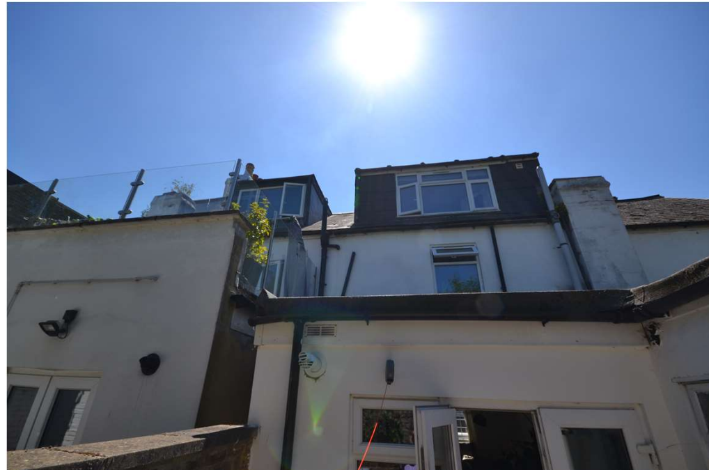
4. View of the rear elevation and neighbouring roof terrace
