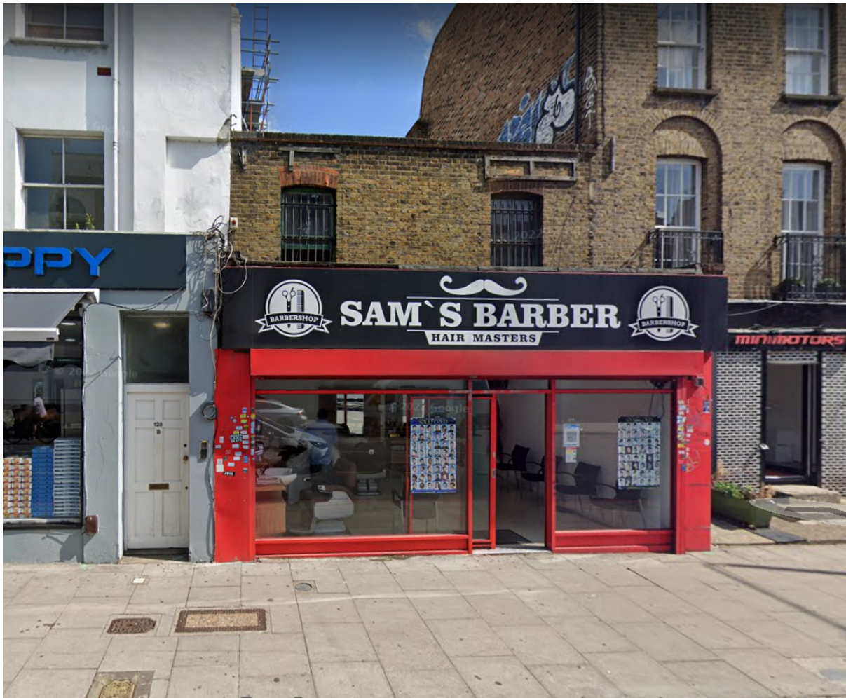
Photo 1 (above): Existing shopfront at 128 Camden Road
