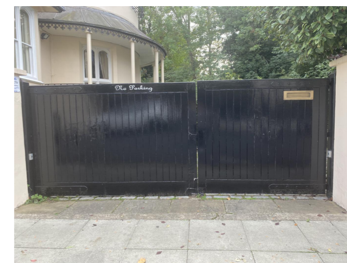
Existing gates - facing Park Village East
