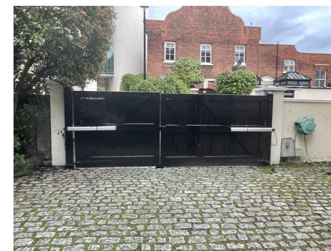
Existing gates - Rear view
