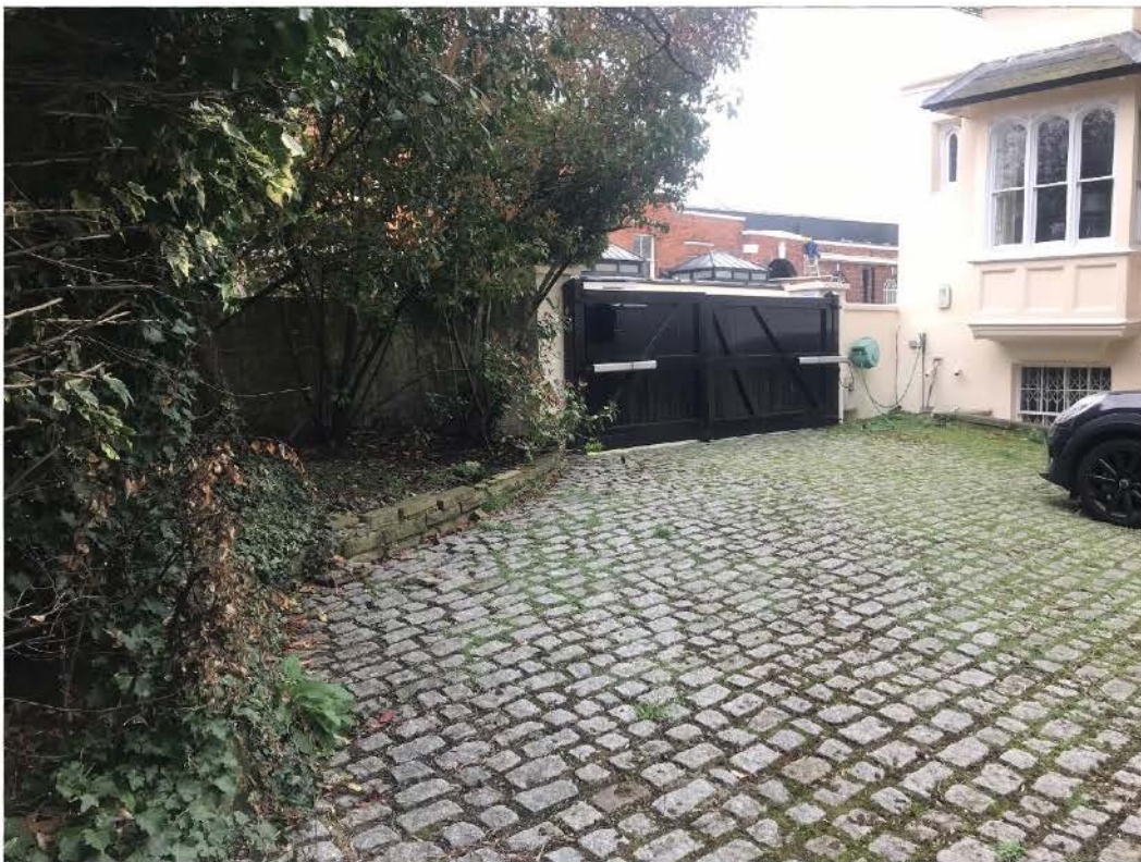
Plate 10: Photograph of the modern granite sets to the parking area directly west of the house
