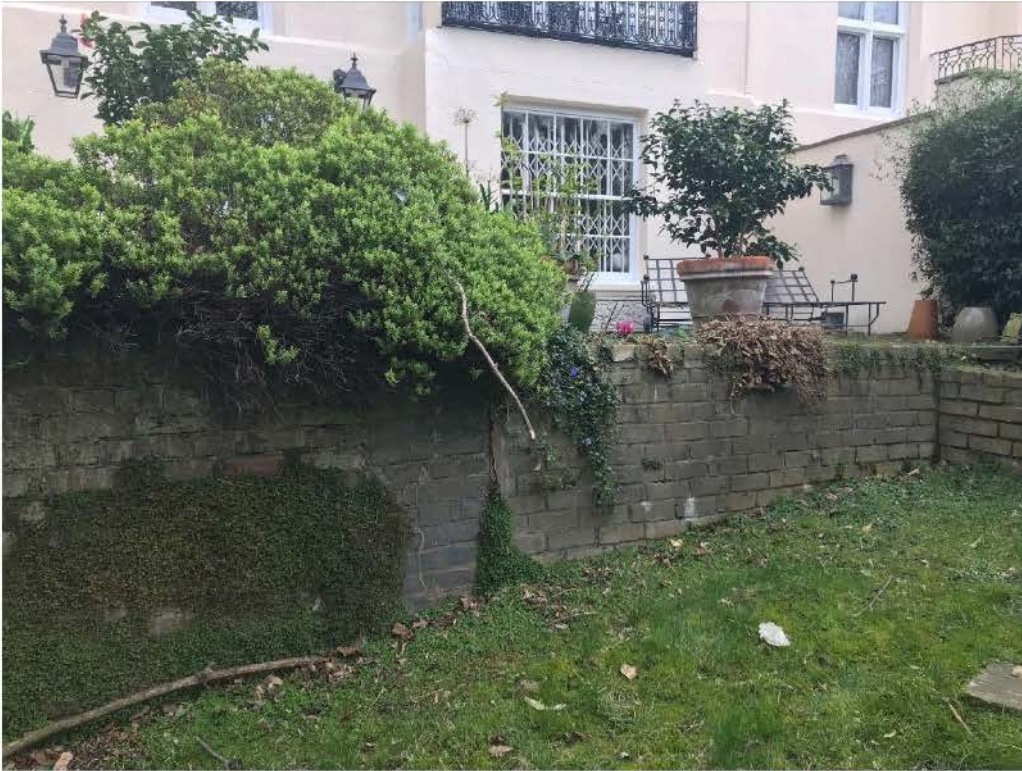
Plate 9: Photograph of the multi-phase brick retaining wall dividing the two principal levels of the garden; the form and style of the brickwork to the right hand side appears to date from 1960-1970
