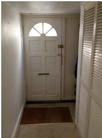
non original front door
