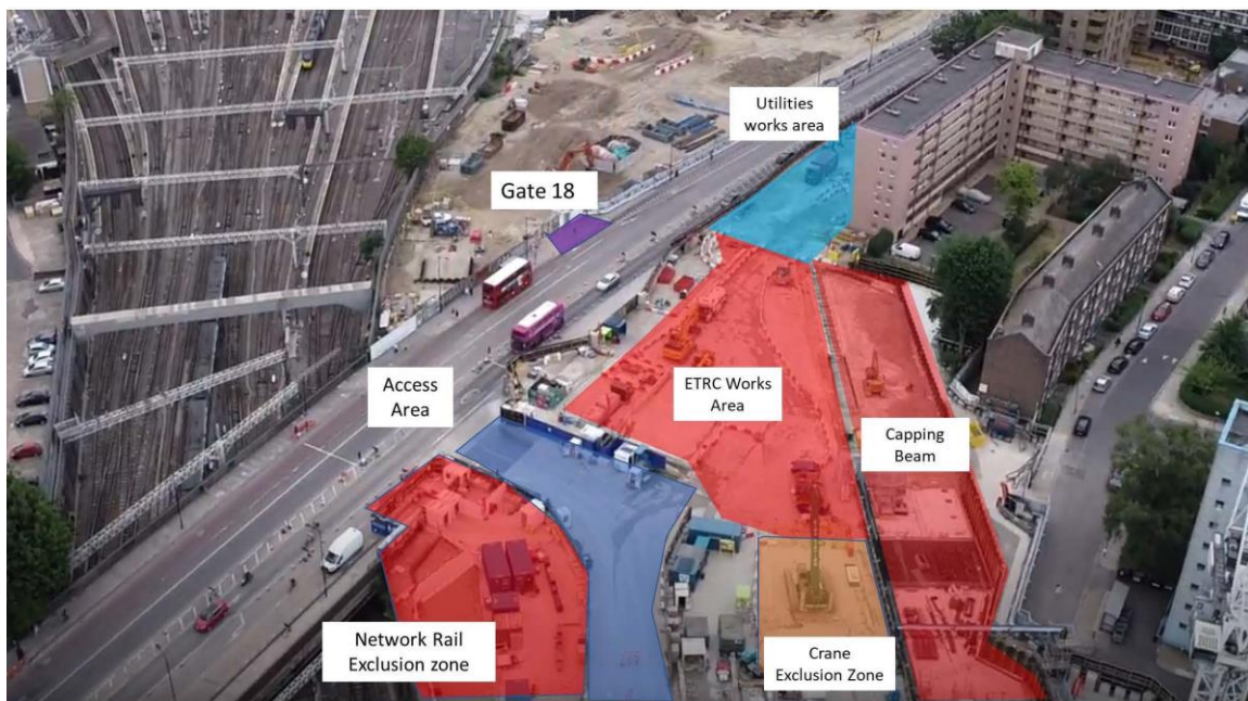
Figure 11: Annotated photograph showing SCS JV worksite (sketch for illustrative purposes).
