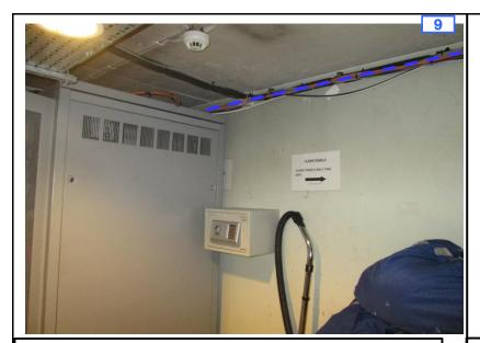
Continue to install new cable within existing galv cable containment towards existing comms cabinet
