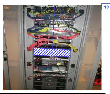
New cable to enter comms cabinet from above and descend into a proposed new craft tray and terminate within.
