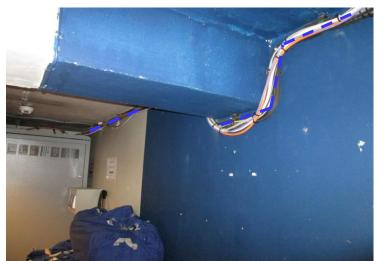
New cable to continue along wall within existing galv containment and navigate towards comms cabinet.
