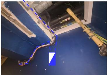
New cable to descend down out of void and run down along existing cable trunking towards proposed new BFP location and terminate within.
