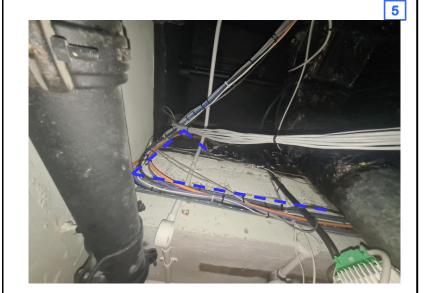
New cable to descend down out of void and run down along existing cable trunking towards proposed new BFP location
