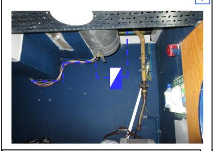
From new BFP install approx 15m new 12F VF cable back up wall and into existing galv containment and navigate towards comms cabinet.
