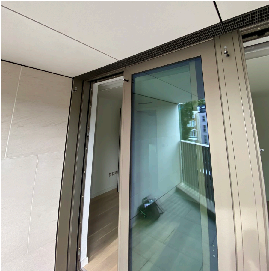
3 Diffusion tubes placed adjacent to MVHR intakes (MVHR not in operation)
