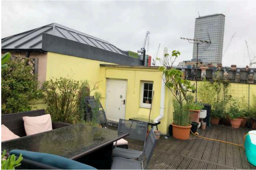
Existing structure at Nos. 34 & 33 - Faux standing seam fibreglass roof at No. 33
