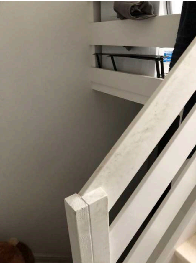
Fig. 5. Existing painted timber balustrade
