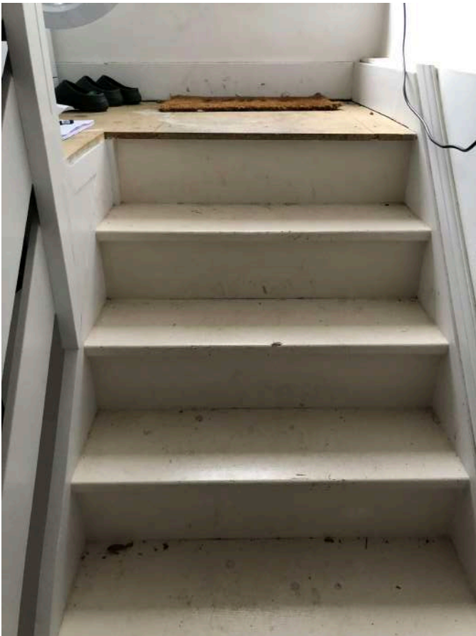
Fig. 6. Existing painted timber stairs and square MDF skirting
