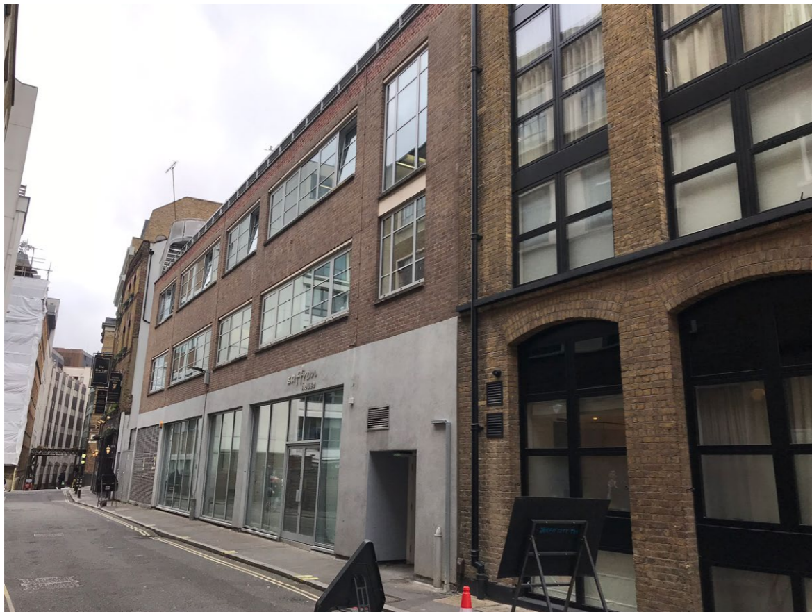
Existing view from Saffron Hill looking South
