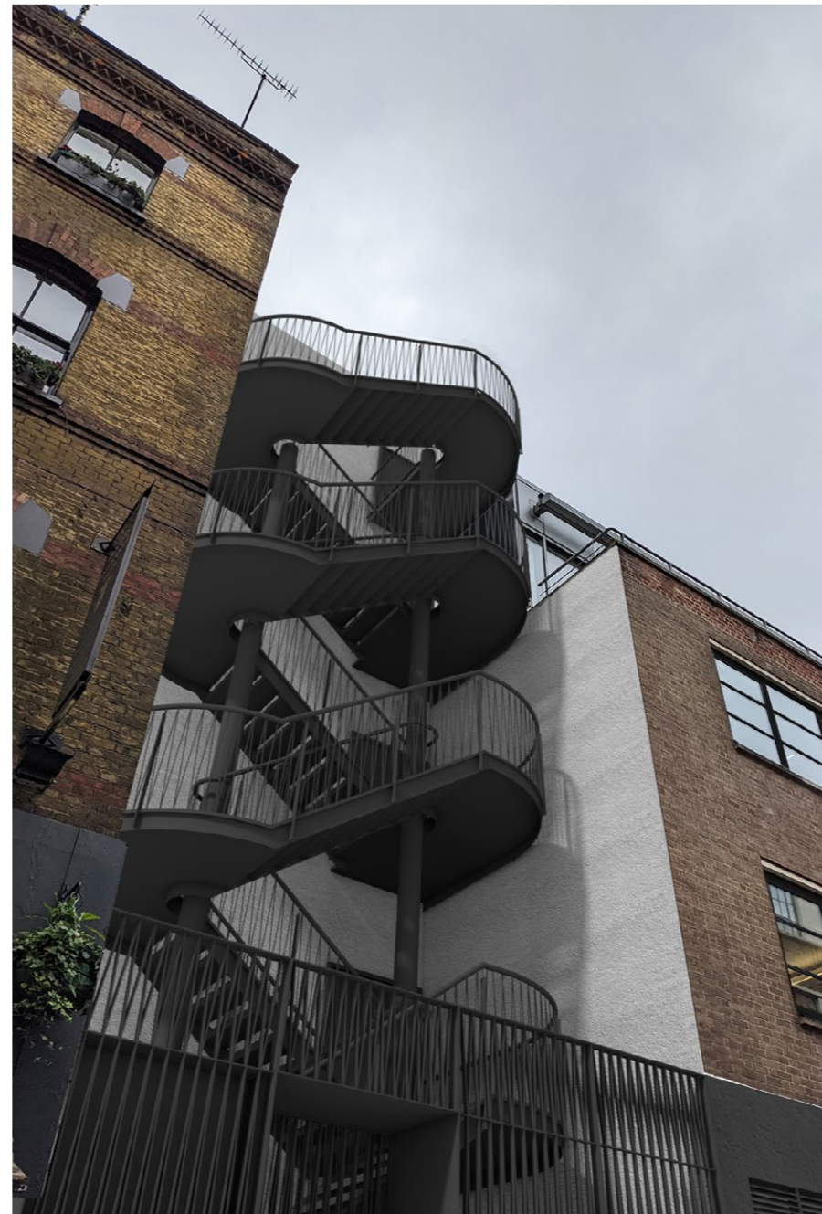
Refurbished stairwell, Saffron Hill
