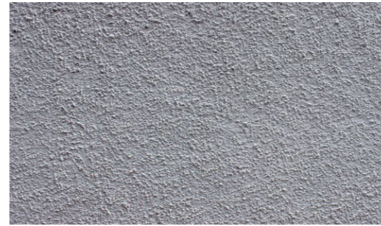
1. Existing render to the interior of the stairwell painted mid grey
