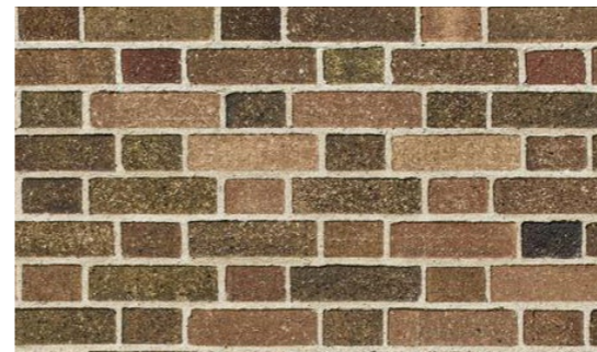
3. Existing Flemish bond brickwork
