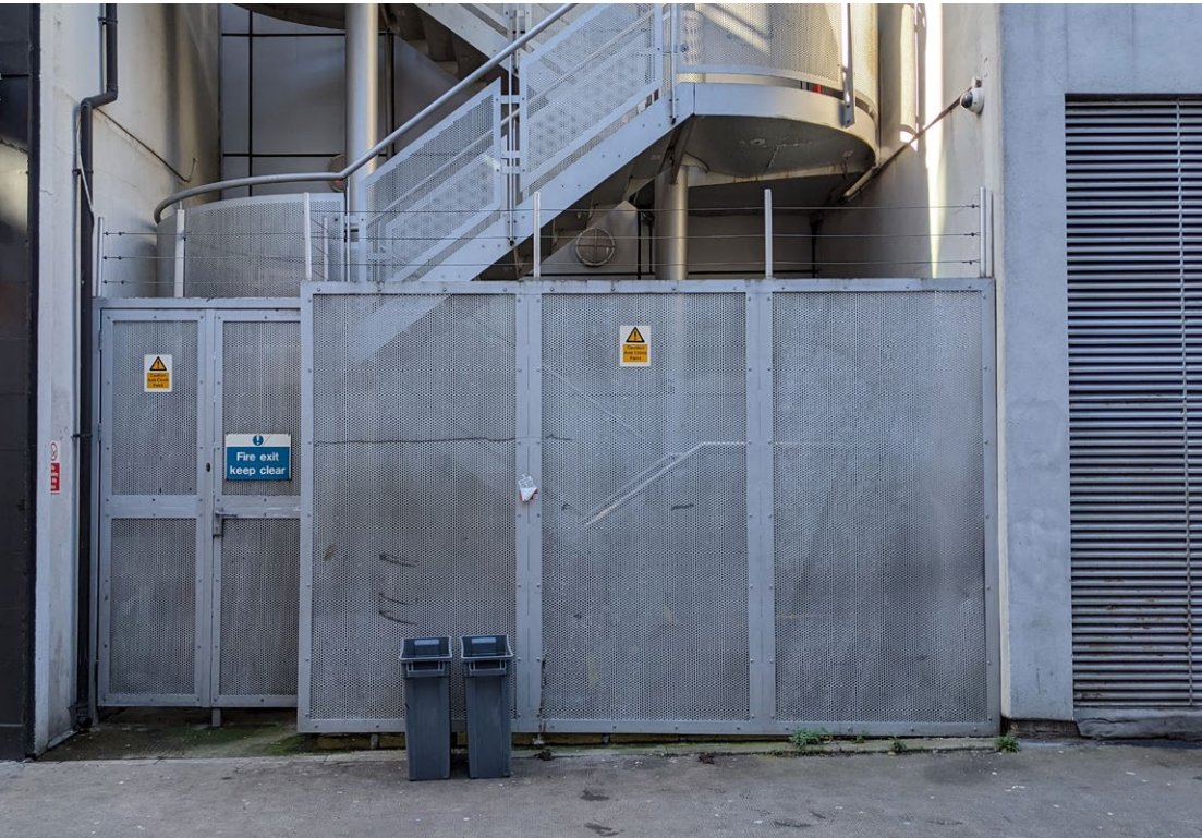
Stairwell screening and escape doors. Metallic cladding behind.
