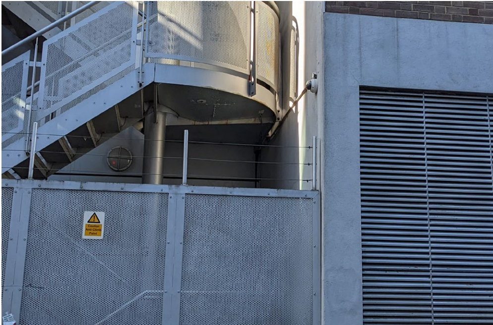
Escape Stair with panellised cladding & original Saffron Hill Frontage. Metallic cladding behind.
