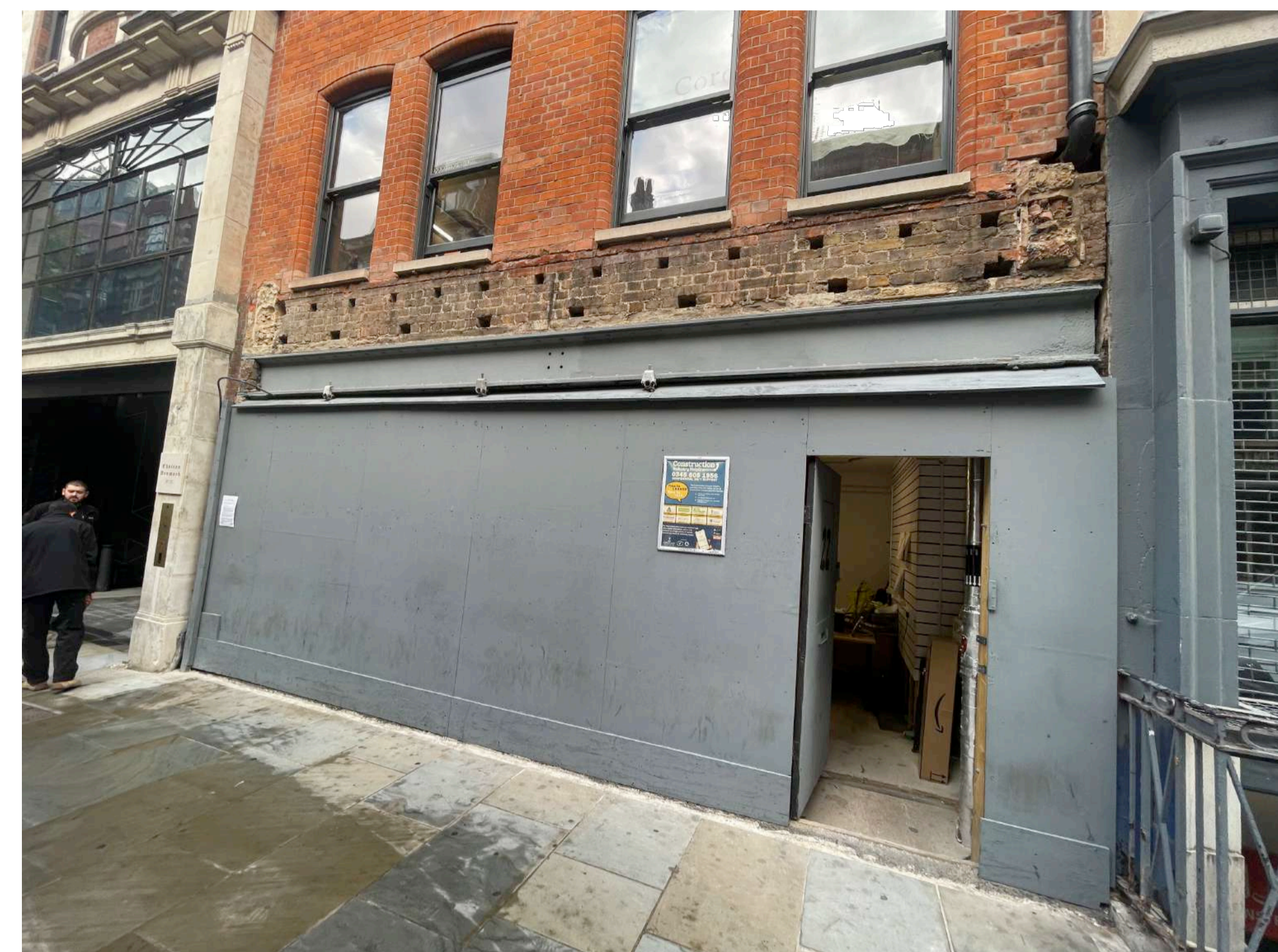
2 Photograph of Existing NTS
