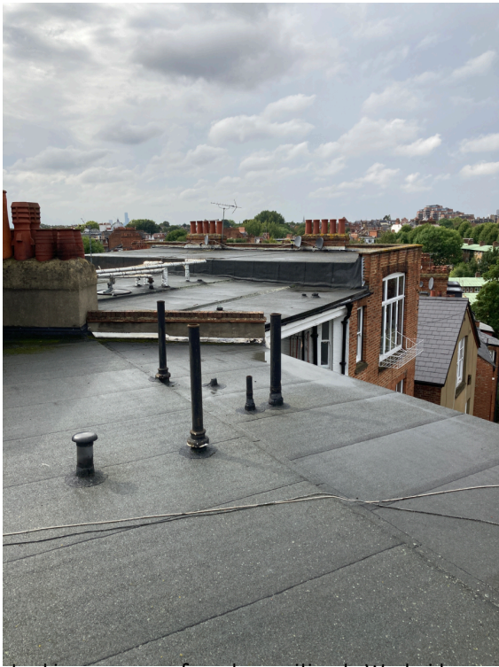
Looking across roof garden position to West side of Stirling Mansions
