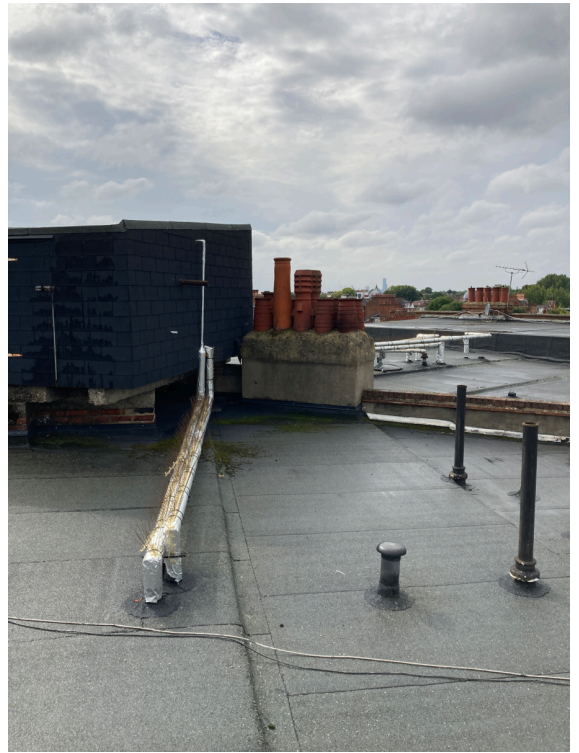
The same showing tank room to be demolished
