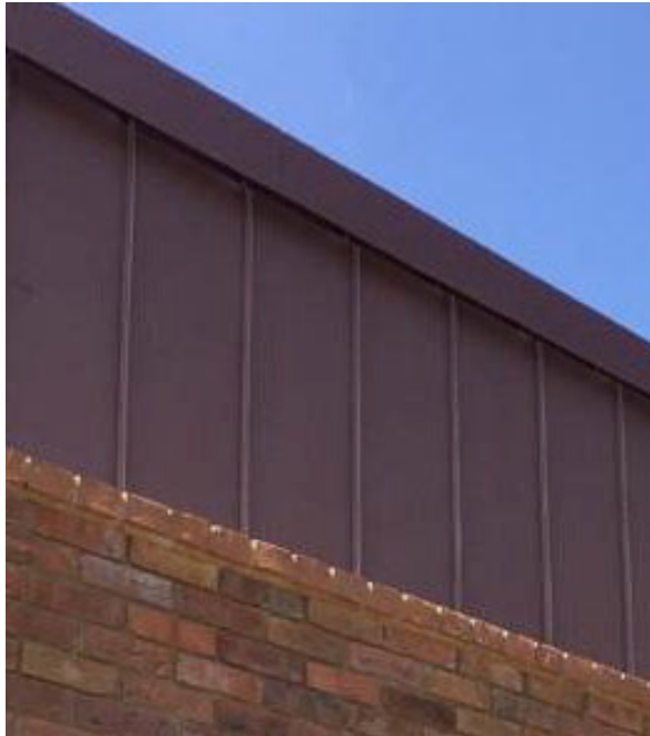
Image of the red pigmented standing seam zinc cladding proposed for use on the plant screens.
