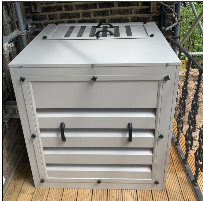
Condenser inside an Acoustic Louvre Enclosure
