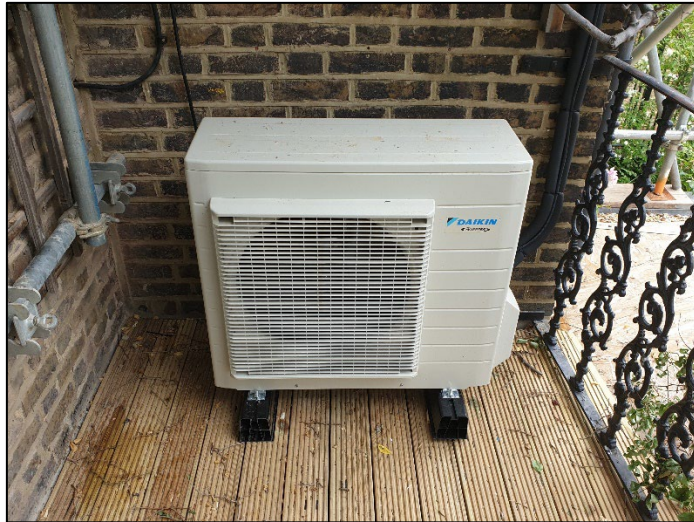
External Condenser Unit
