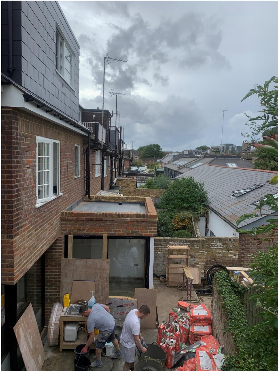
Image 2 (above): Photo on roof of extension looking south
