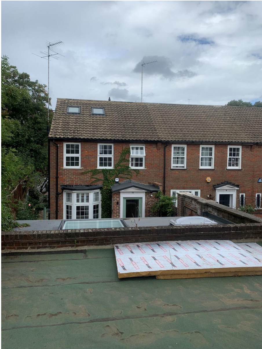
Image 4 (above): Photo from roof of extension looking North
