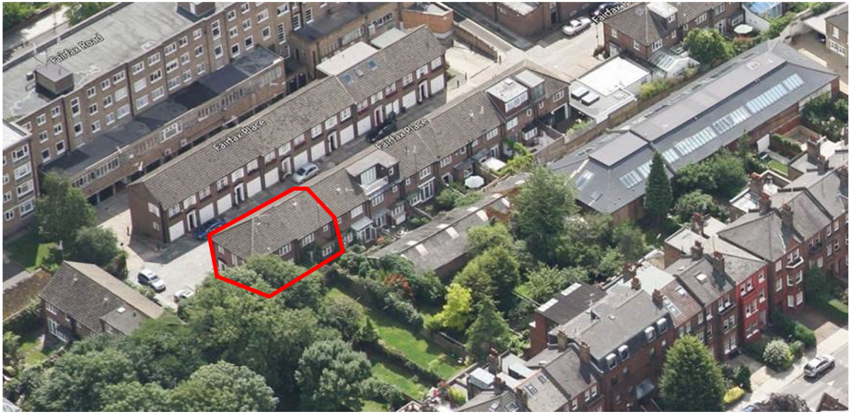
Image 1 (above): Photo of south facing rear elevation
