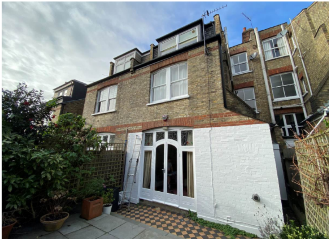
Picture 3: Rear elevation
