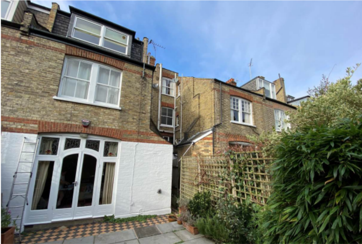
Picture 4: Rear elevation & adjacent No39
