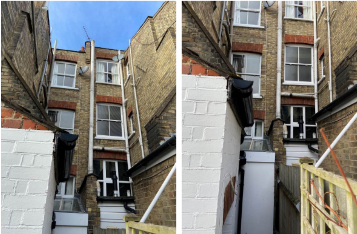
Picture 5: Rear elevation & adjacent No39
