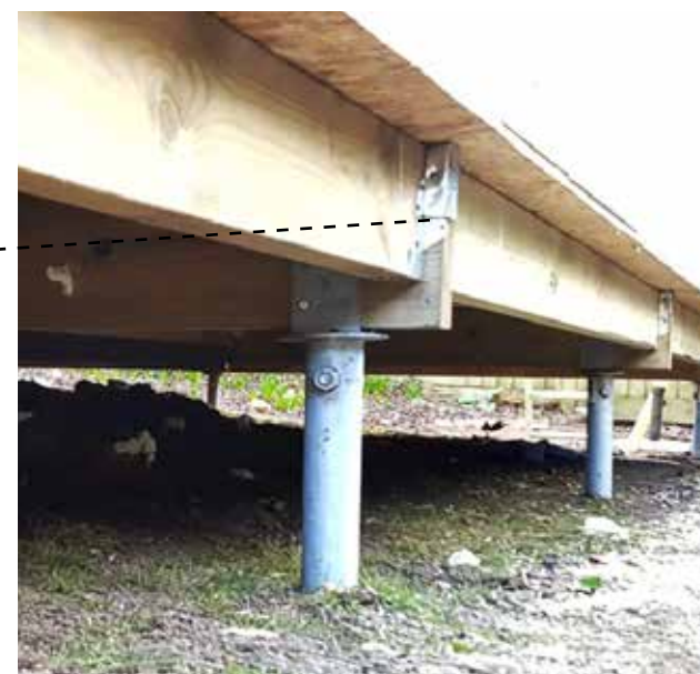
FIG. PROPOSED SCREW PILE
