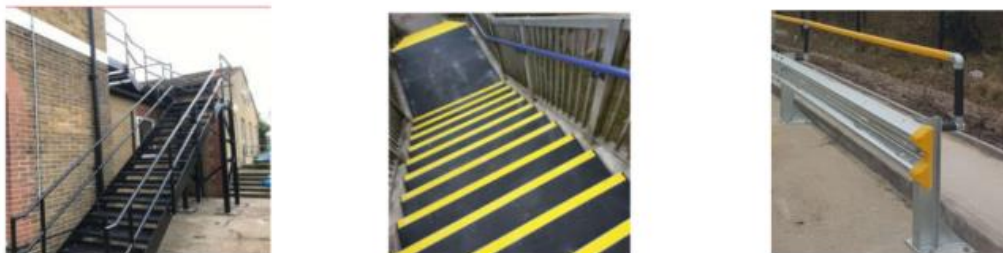
Figure 3-6 - Proposed materials: painted steel stairs, yellow tread nosing, crash barrier
