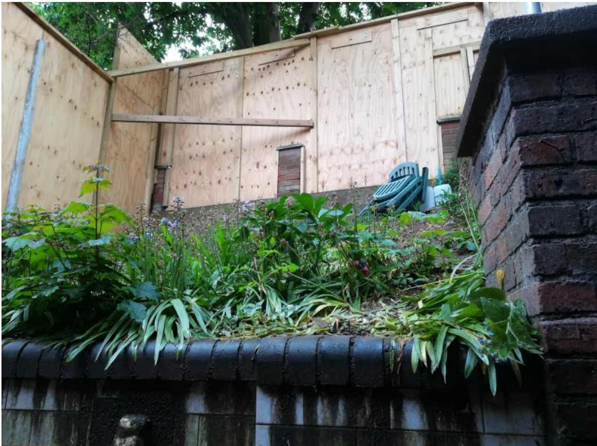
Photo 7: Looking up towards the area where the bin and cycle store is proposed, showing the level rise (with T2 behind the timber hoarding).
