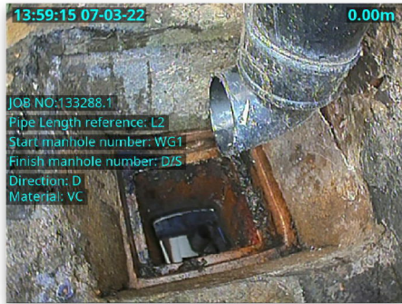
Fig 4.1: Damaged Gully
