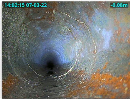
Fig 3.1: Line 2 Cracking
