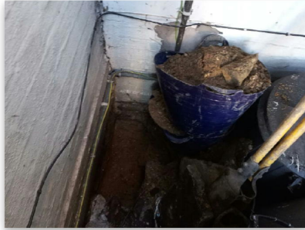
Fig 2.1: Attempted Trial Hole 2 Location
