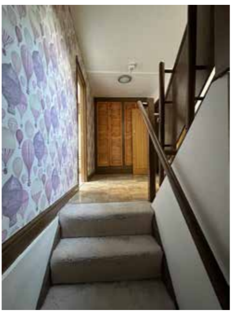
1. original stair treads covered in carpet, original balustrade + handrail painted over
