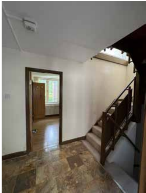
5. non-original wall + door + frame, original sliding door + track not present
