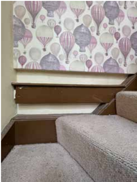
4. non-original wall blocking stair from kitchen below, original stair structure intact
