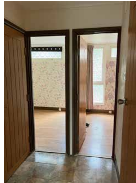
1. floor to ceiling sliding doors + track missing, replaced with wall + two swing doors/frames
