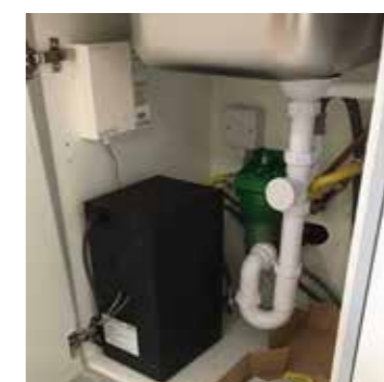
"Plumis" Mist System Water Pump (connects to mains water supply)
