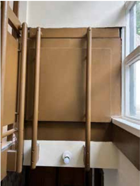
5. original balustrade + hand-rail painted over, connections + details still present
