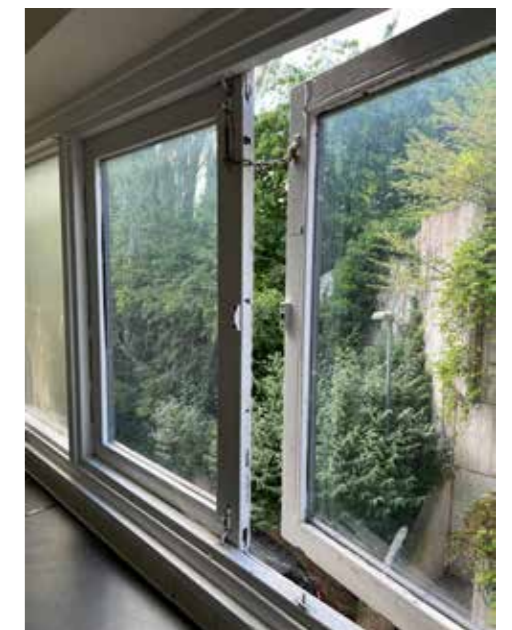
6. original windows painted white internally, and in significant state of disrepair
