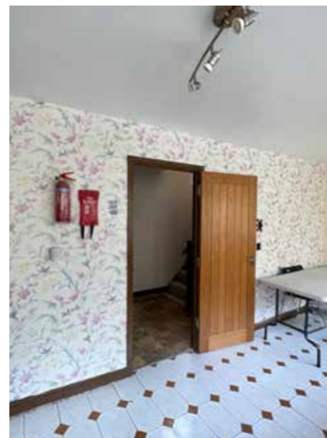
4. non-original wall + door + frame, original stair balustrade no longer present
