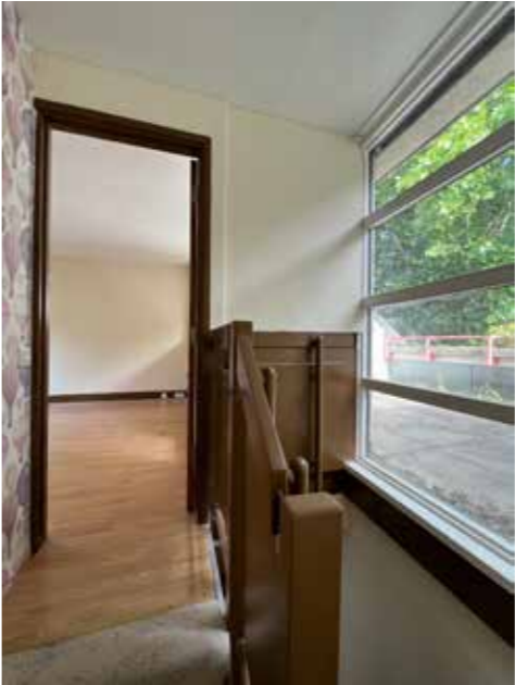
2. non-original stud wall + door + frame built behind original balustrade
