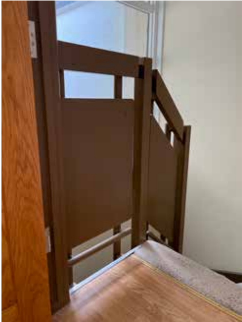
3. original balustrade + handrail painted over, note non-original floor finish
