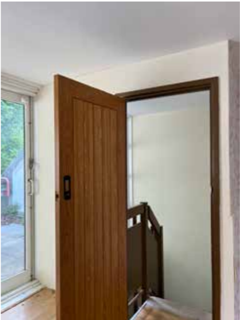
5. non-original wall + door + frame to stair, concealing original balustrade
