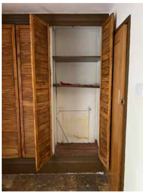
3. original asbestos service void access panel to be replaced with modern equivalent
