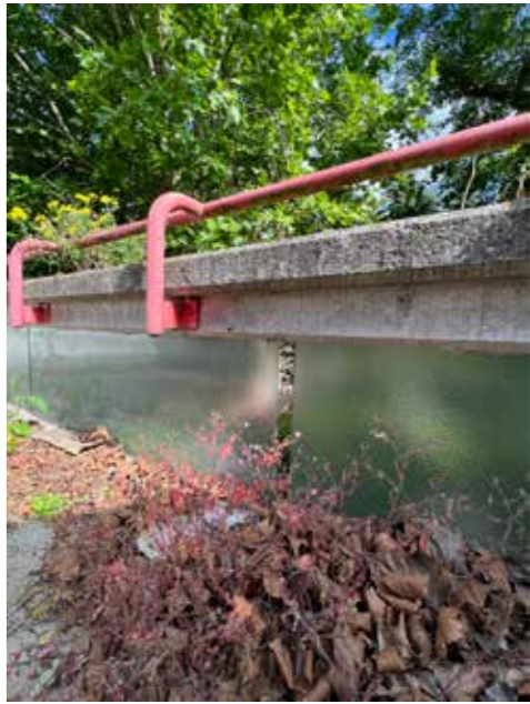
3. original handrail intact, paint faded/damaged, original glass screen still present
