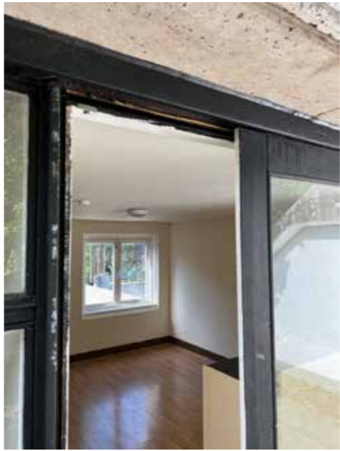
2. exterior sliding terrace window in original finish/colour, unaltered, but in state of disrepair
