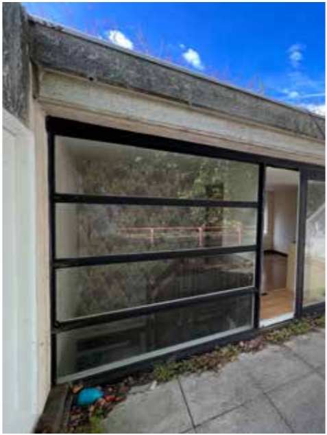
1. exterior fixed terrace window in original finish/colour, unaltered, but in state of disrepair
