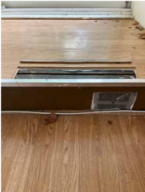
4. original raised plinth covered over - original material intact underneath, albeit painted
