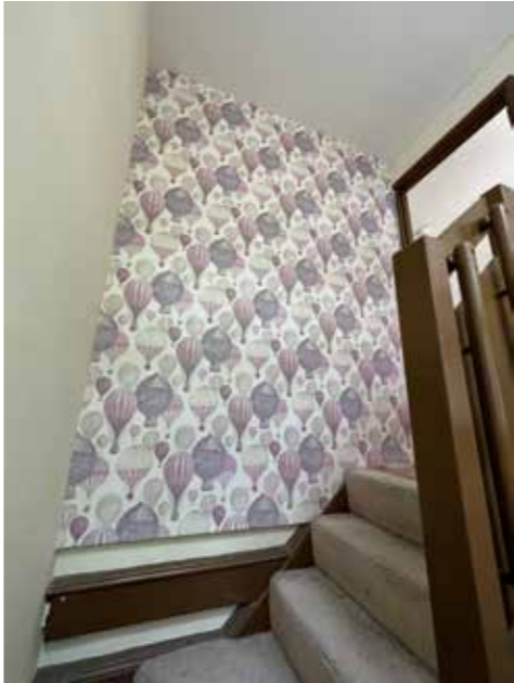
1. stud wall built on top of original parapet wall, separating living space from stair
