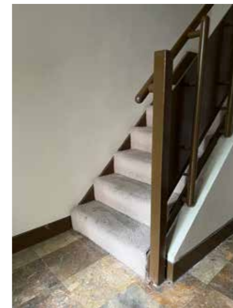
5. original stair treads covered in carpet, original balustrade + handrail painted over
