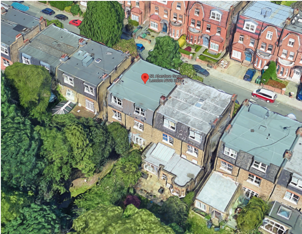
2. Aerial view - rear
