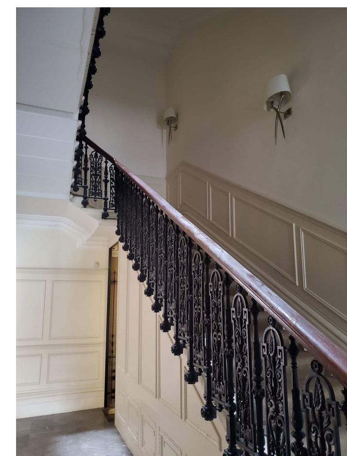
Reference photograph of existing staircase panelling
