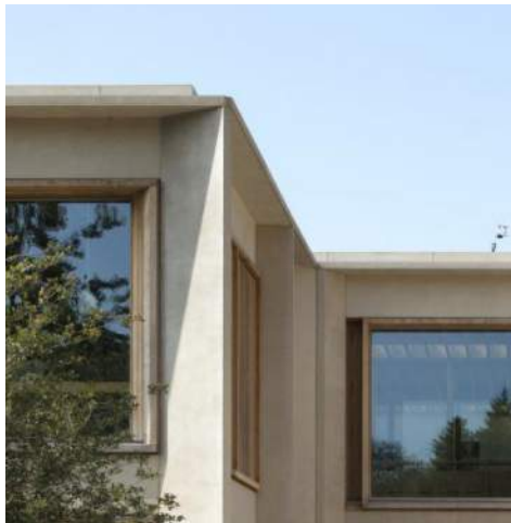
1. Pale stone with lime pointing
