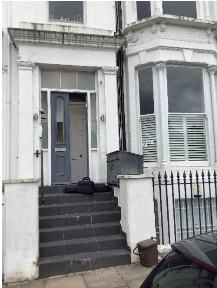
Front elevation of main property
