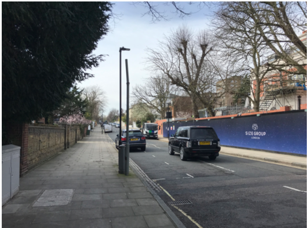
View of Queens Grove.
