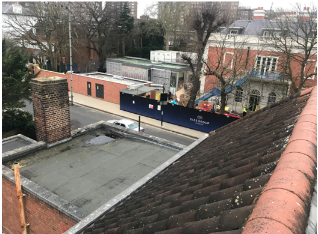
View towards 75 Avenue Road taken from the roof of 71 Avenue Road.
