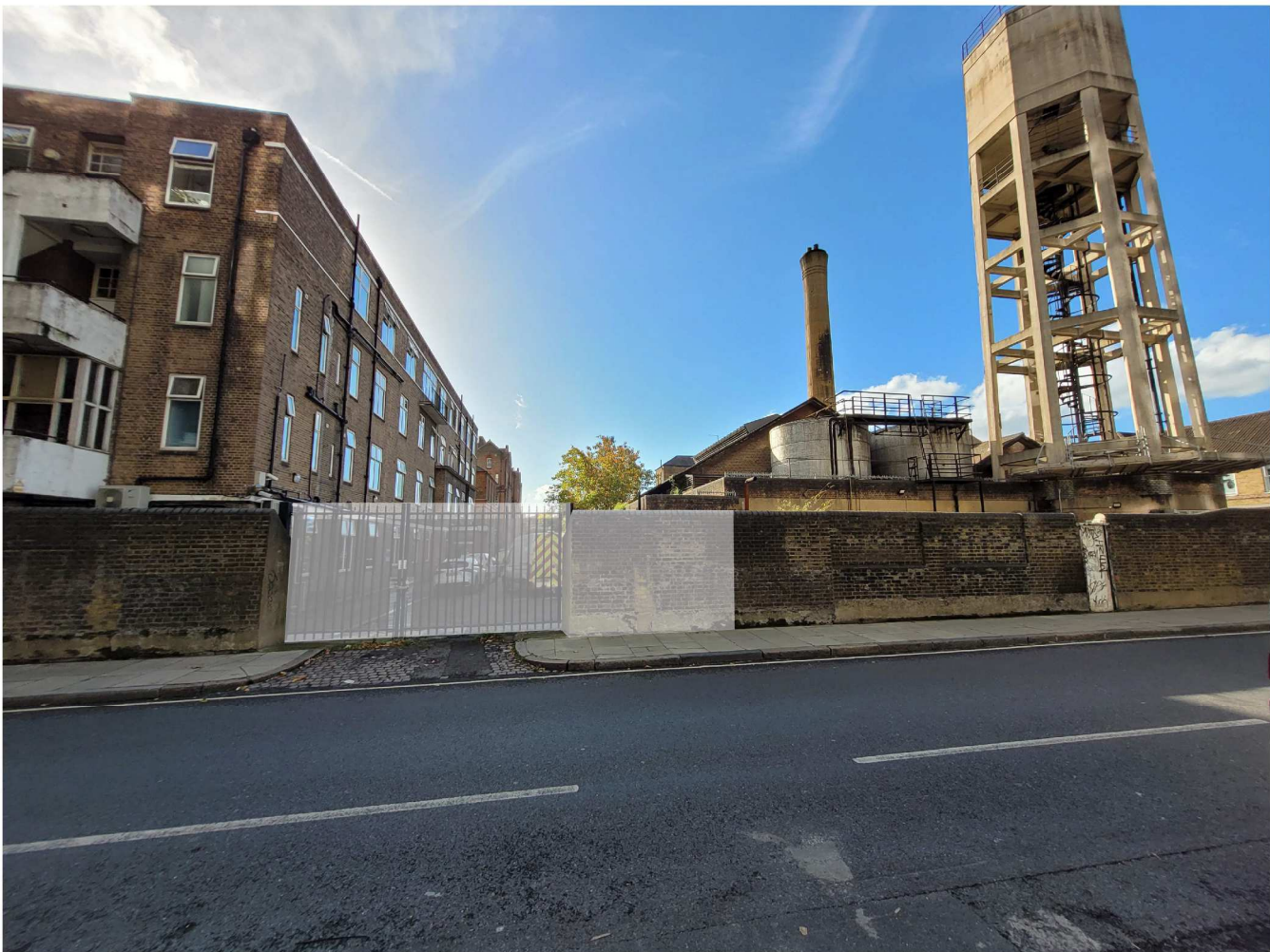
Temporary footway crossover 1
