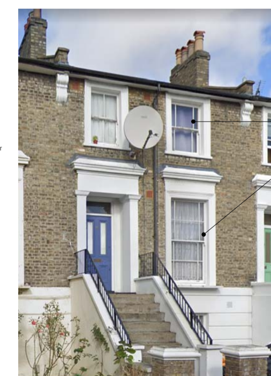
Reference Photo - Front elevation of neighbouring property.
