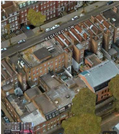
Figure 19 The rear façade of the Bedford Row frontage block.
