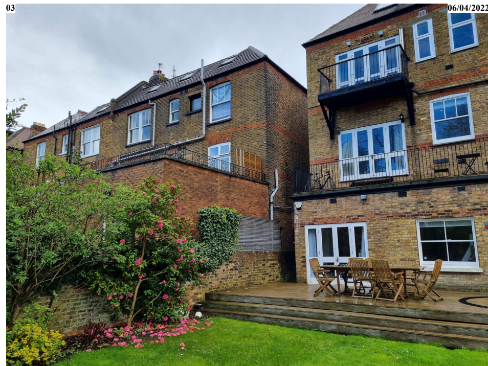
- No.58 Canfield Gardens rear elevation seen from No.60 rear garden.
