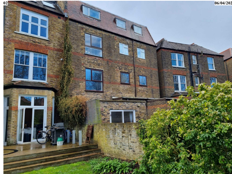
- No.62 Canfield Gardens rear elevation seen from No.60 rear garden.
