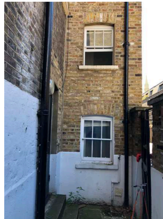
Site Photo - Ground Floor. Rear yard looking outrigger.
