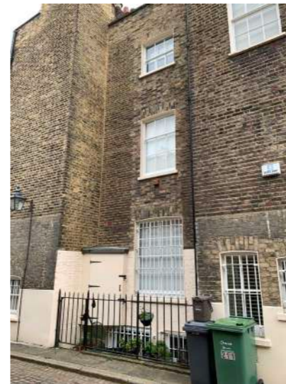
New sash windows at 211 Albany Street rear elevation.
