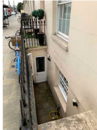
Door arrangement under 209 Albany Street entrance.
