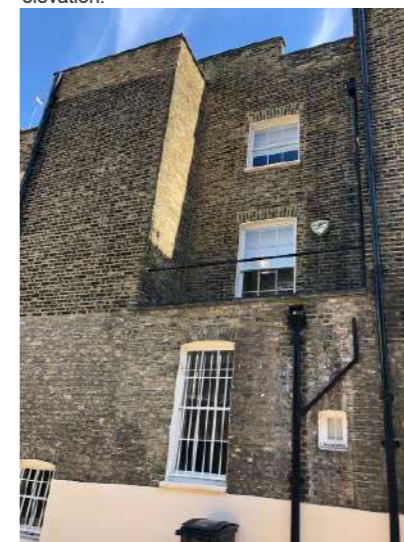
Higher and fully closed rear yard at 213 Albany Street.
