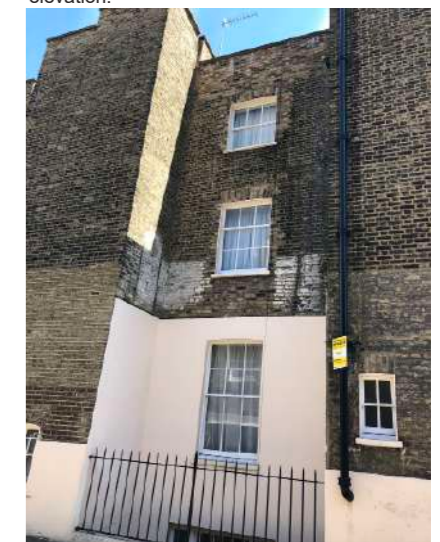
Railing at rear yard at 217 Albany Street.
