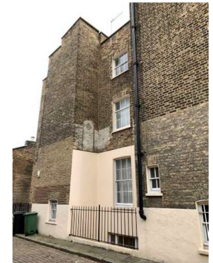
New sash windows at 217 Albany Street rear elevation.
