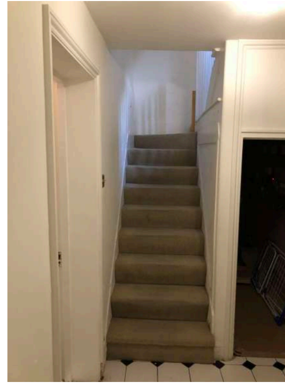
Site Photo - Basement. Stairs to Ground Floor.
