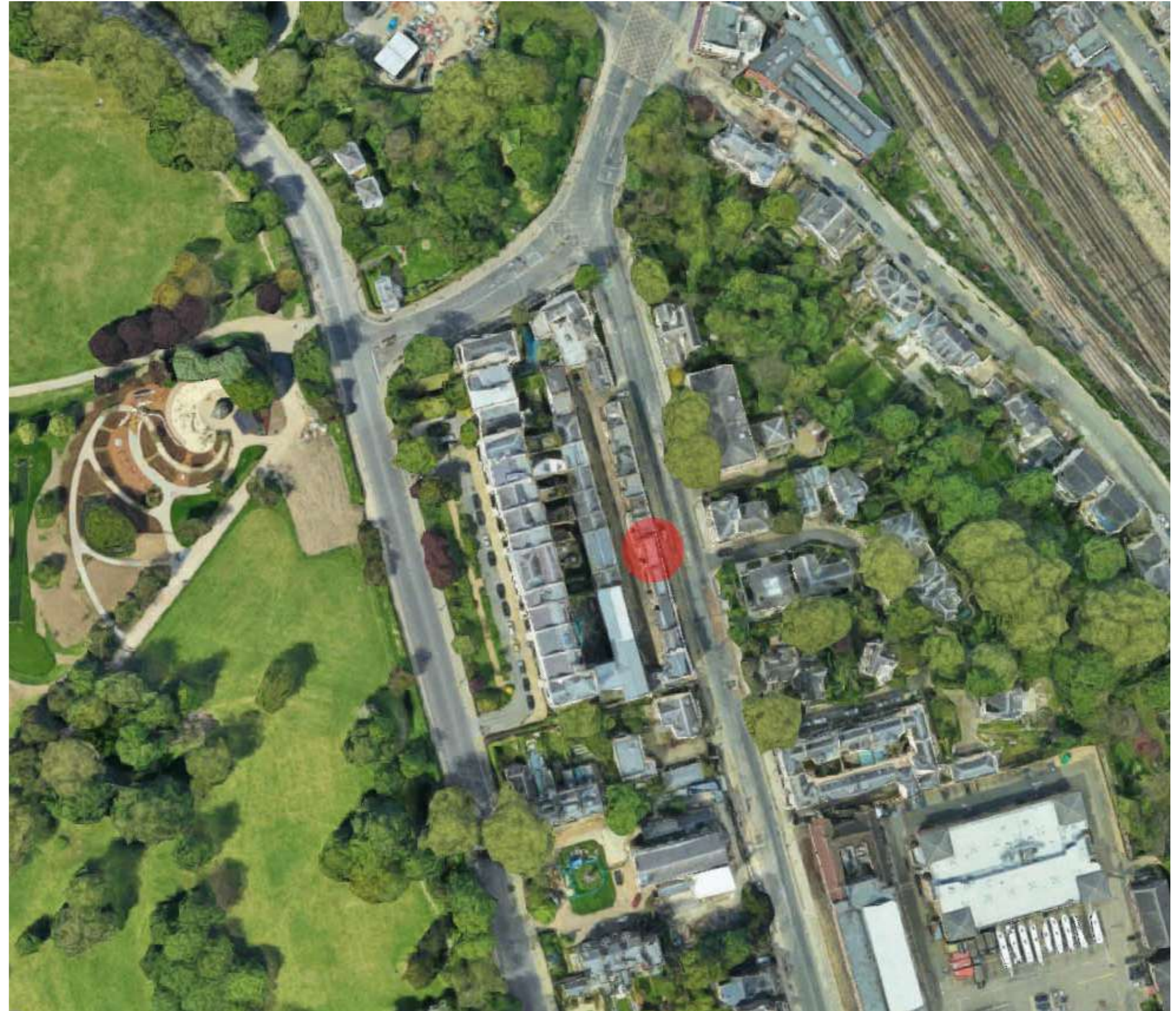
Aerial Photo - 205 Albany Street
