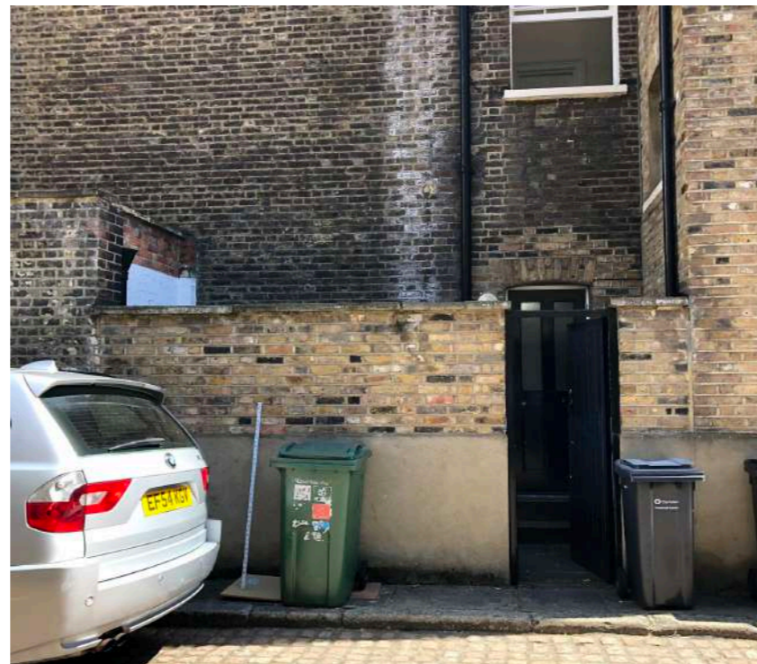
Site Photo - Existing rear elevation from Gloucester Gate Mews
