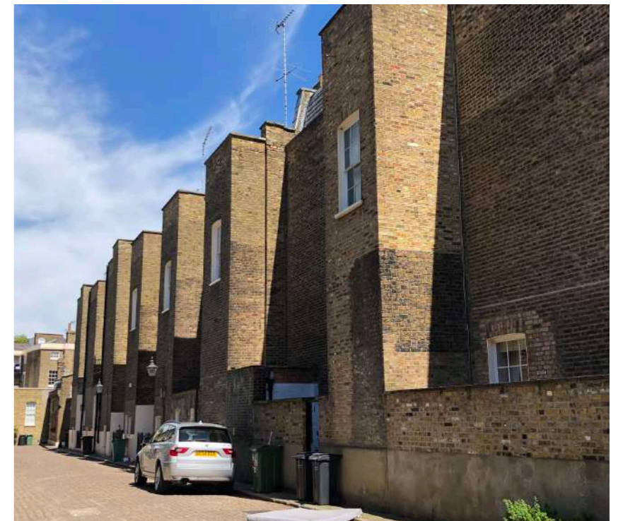
Site Photo - Existing rear elevation from Gloucester Gate Mews and surroundings
