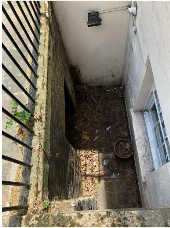
Site Photo - Basement. Light well.
