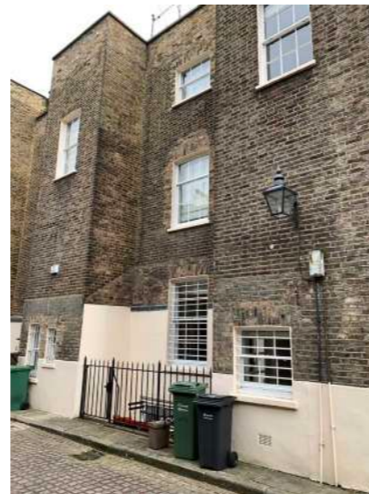
New sash windows at 209 Albany Street rear elevation.
