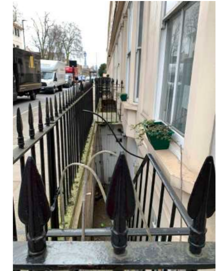
Door arrangement under 217 Albany Street entrance.
