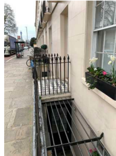
Door arrangement under 211 Albany Street entrance.
