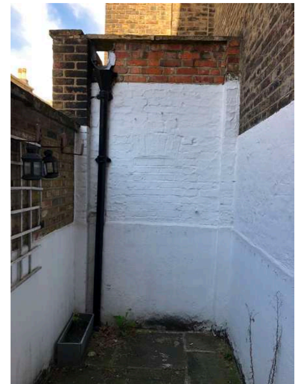
Site Photo - Ground Floor. Rear yard looking extension.
