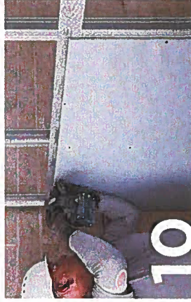
10 For angles and double stud bay horizontal beam joints use a GypWall DSI Flying Stud to Partitioning Centres.
