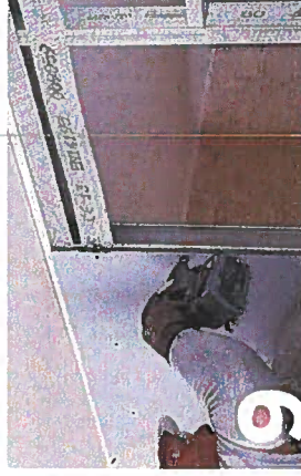
9 Use British Gypsum Drywall Screws to fix GypWall plasterboard or Glasroc specialist boards to GypWall framework.
