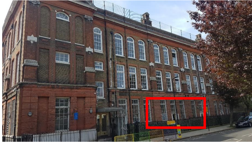
Photo 1: PCPS Centre to be located in former ground floor classrooms
