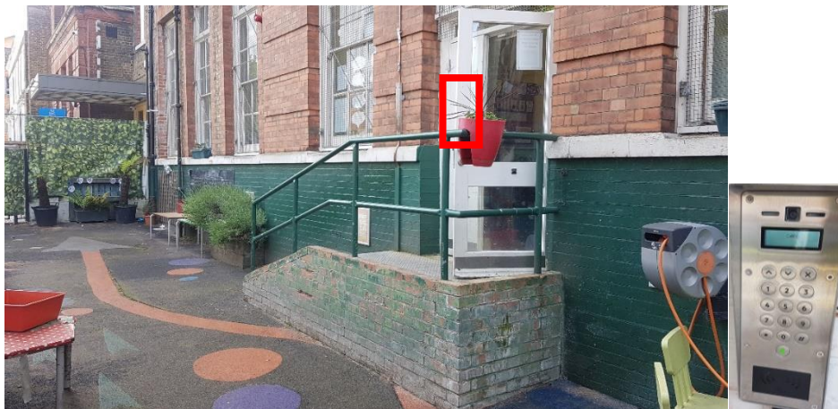
Photo 3: Proposed door access entry panel
