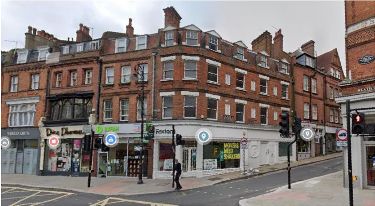
47 Heath Street (Foxton's Building) – Heath Street/Holly Hill elevation
