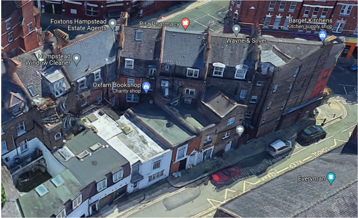
Holly Bush Vale elevation (47 Heath Street = white painted building)
