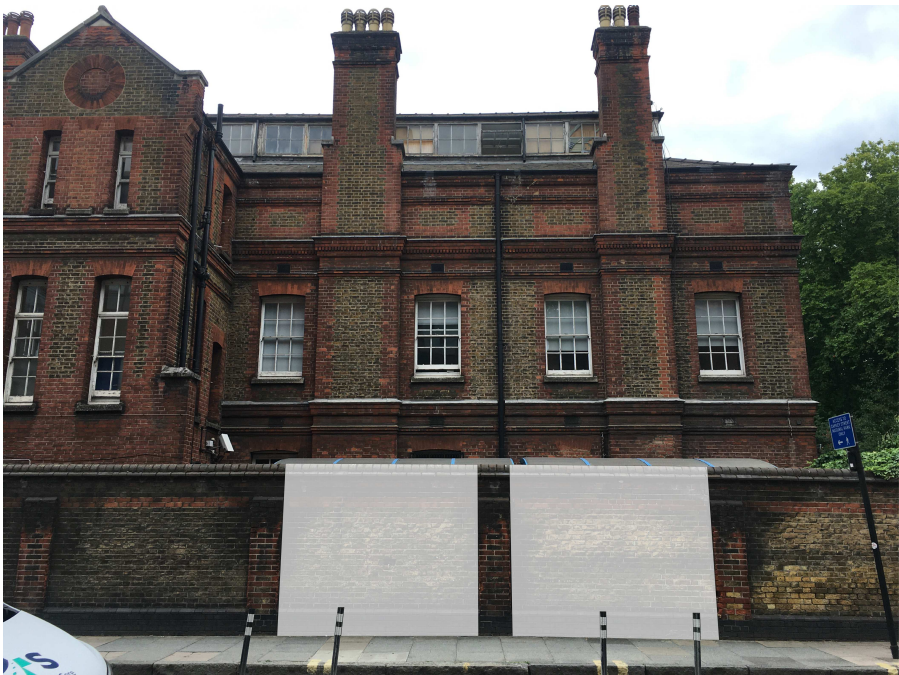
Existing site photograph with highlighted areas showing the sections that will be demolished carefully with the bricks being saved to be used when the wall is rebuilt
