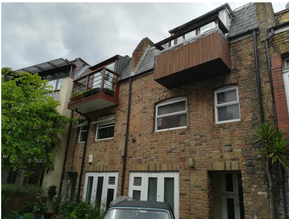
Existing balconies to no. 7 & 8 Eglon Mews
